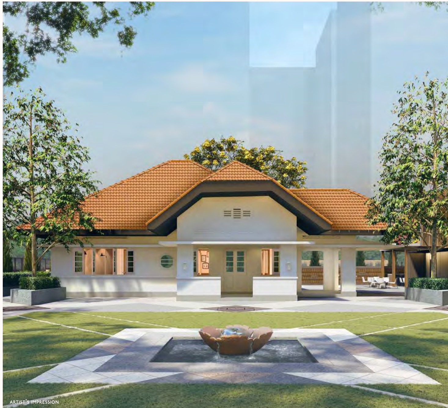
Timeless memories await at the refurbished Thiam Siew House. The clubhouse features a decorative wall that preserves the property's Marseille roof tiles, a mid-19th century innovation,
